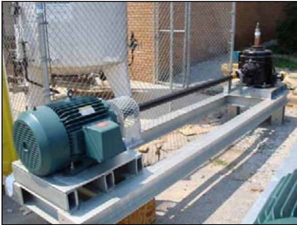
**Figure 1: Typical Fan Drive Arrangement**
