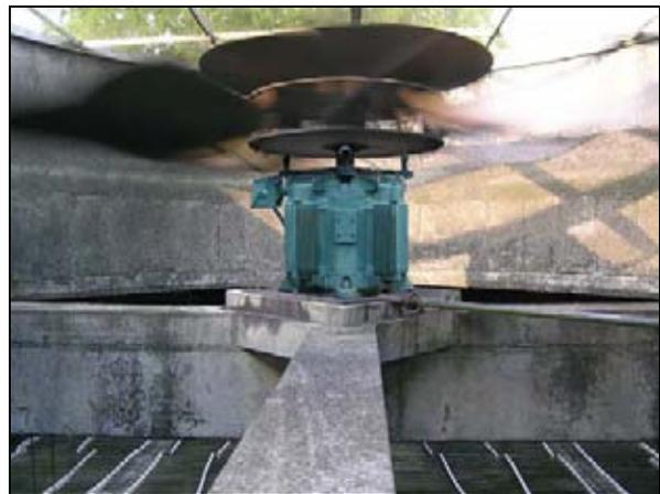
**Figure 7 – PM Motor Installed in Place of Gearbox & Driveshaft**
