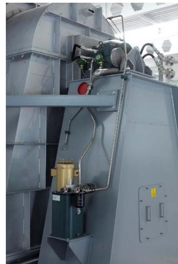
**Figure 7.** Hydrodynamic fan bearing configured for circulating oil.
