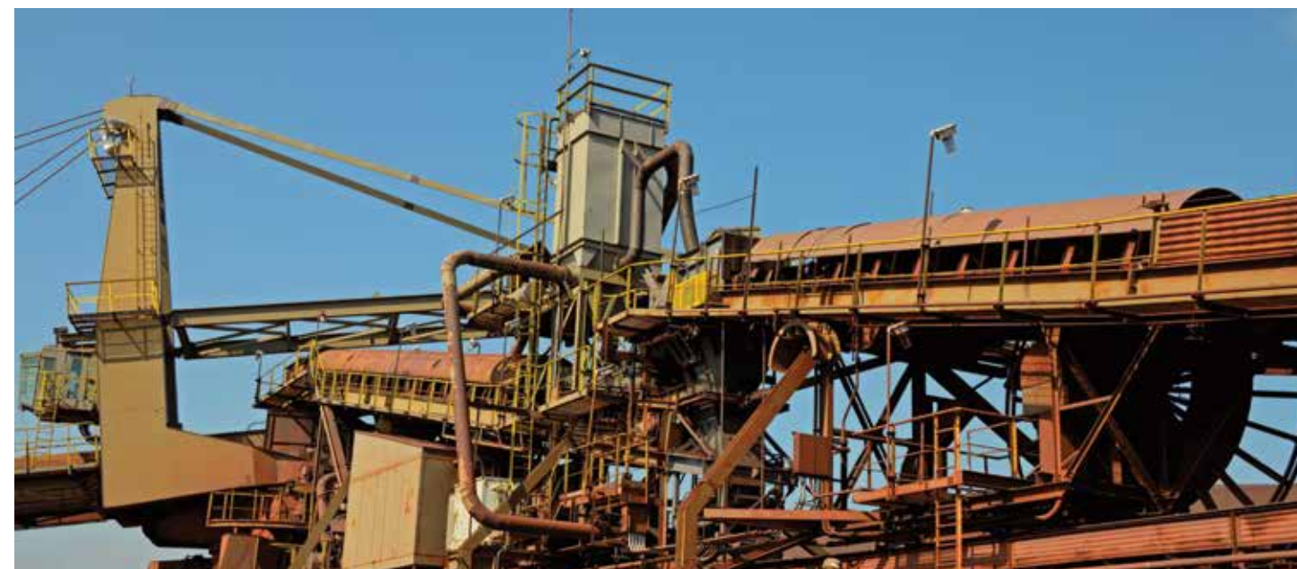
When the maintenance team spent 48 hours to remove and replace a failed split cap SAF-style bearing, maintenance foreman Ron Davenport knew there had to be a better bearing solution. While Davenport was skeptical that a bearing could be installed or removed quickly and easily, he became a believer in Baldor's Dodge Hydraulic ISAF bearing after he and his team installed the bearing in less than 15 minutes.
