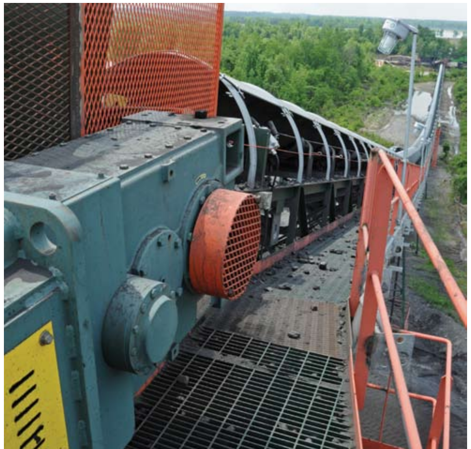
A 210K MagnaGear XTR was selected to operate this 1,197-foot-long conveyor, with an 86-foot lift. This conveyor moves coal from the river barge to Armstrong's prep plant.
