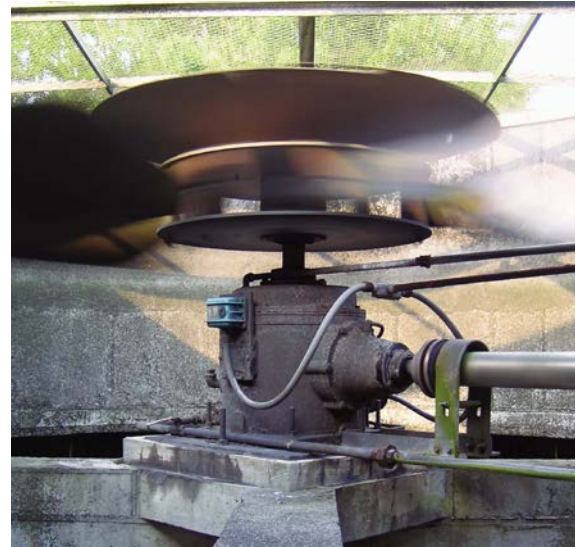
A typical conventional fan drive arrangement of a gearbox mounted under the fan.
