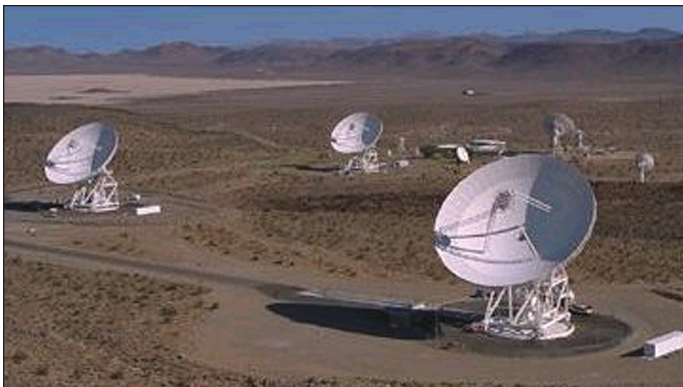
"Courtesy NASA/JPL-Caltech." JPL Goldstone, CA Complex, 34M Beam Wave Guide (BWG) Antennas
