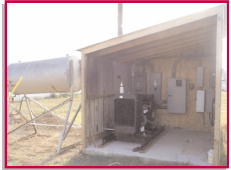
Richmond Ranch standby generator installation
