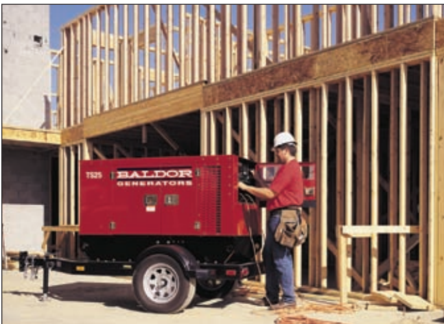
Baldor TS25T providing power for framers and roofers at a new construction site.
