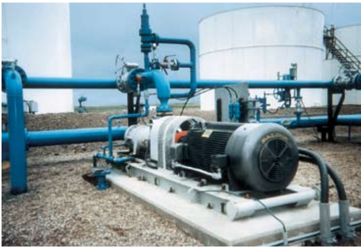
This 450 Hp Baldor pump motor transfers oil from tank to tank. Our line of pump motors includes single or three phase jet pump, square flange, close-coupled, and P-Base vertical solid shaft pump motors. The motors are stocked in totally enclosed fan cooled, open drip proof, and many explosion proof ratings.
